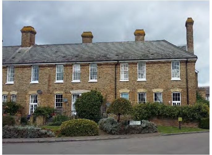
Redeveloped former workhouse along A291 Canterbury Road
