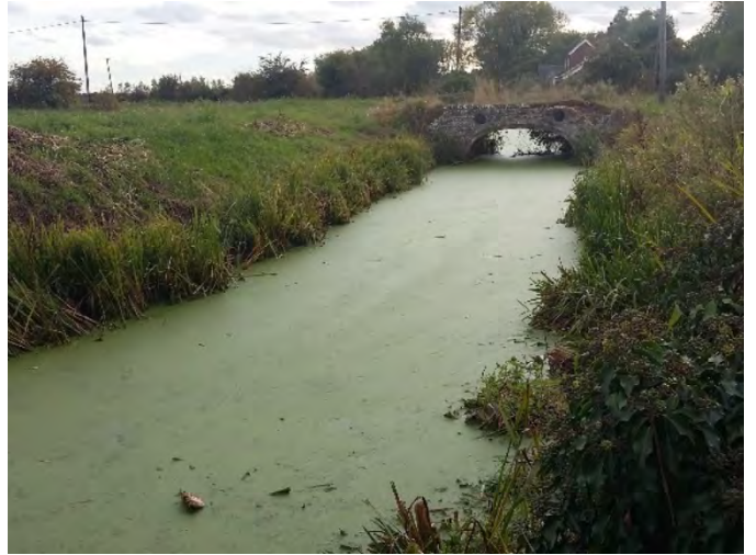
Brick bridge crossing North Stream north of Marshside
