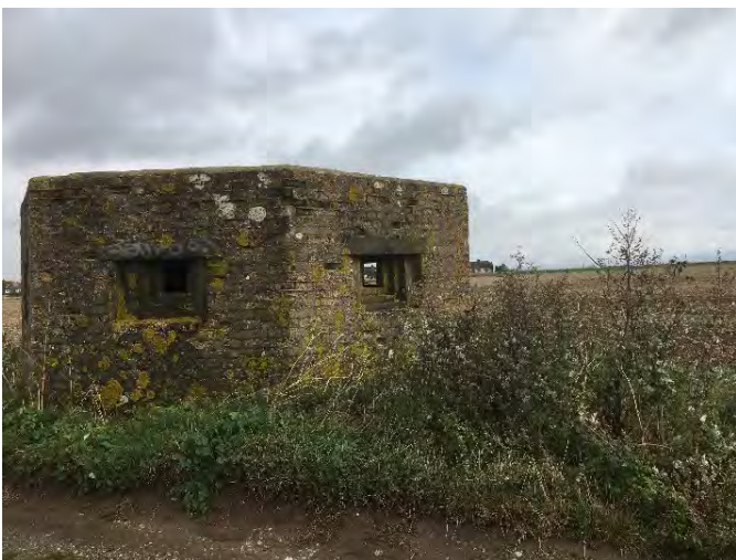
Pillbox along Adisham Downs Road, part of WWII defences
