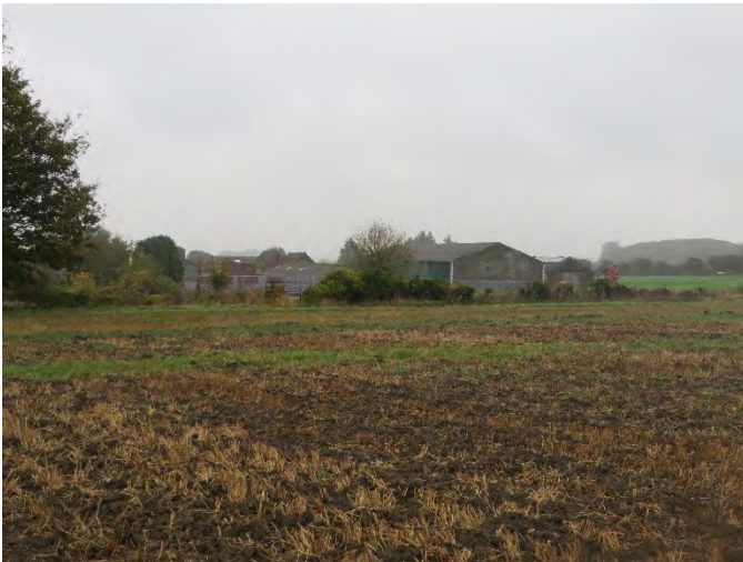
Large agricultural buildings / structures visible across farmland
