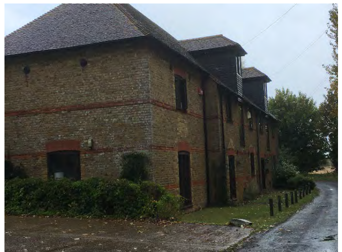
Converted farm buildings forming part of the Conservation Area at Bossington
