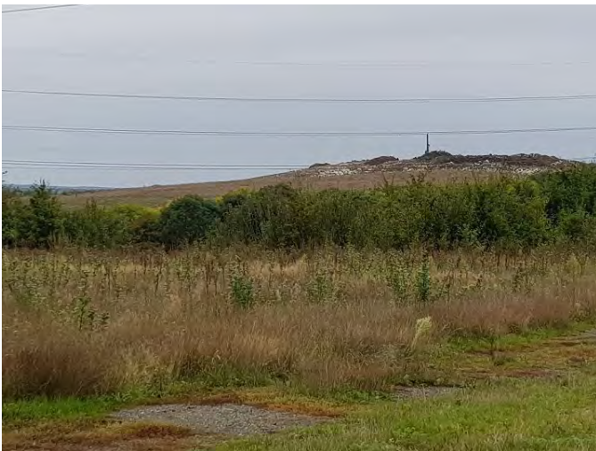
Shelford landfill and gas recovery
