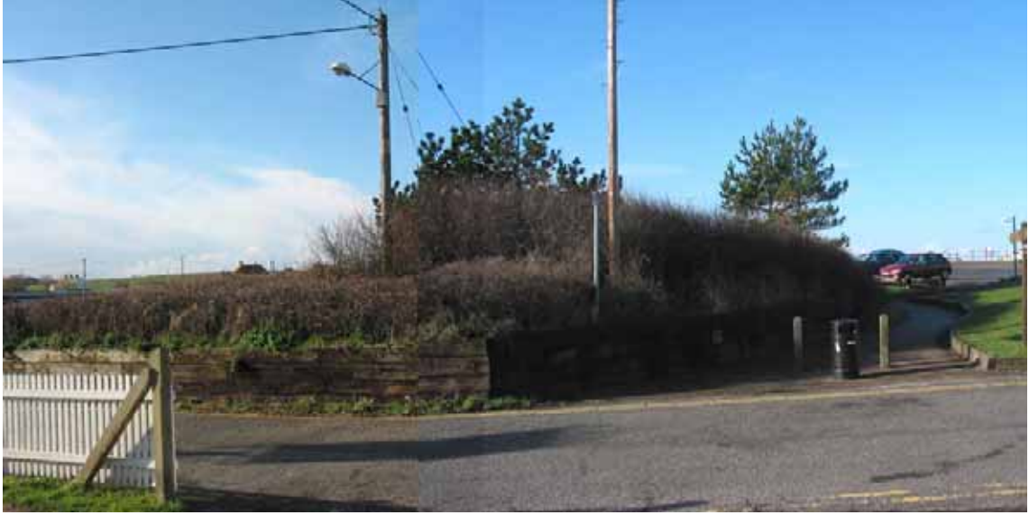
Existing edge. Retaining sleeper wall and shrubby edges restrict free access and obscure views into space
