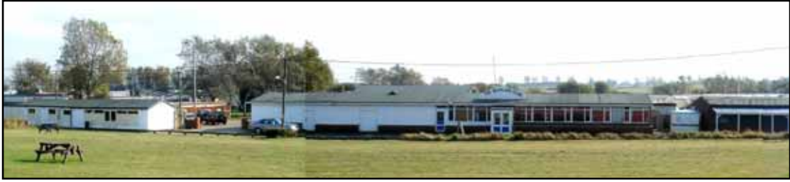
Existing cafe, shop, arcades and Reculver club
