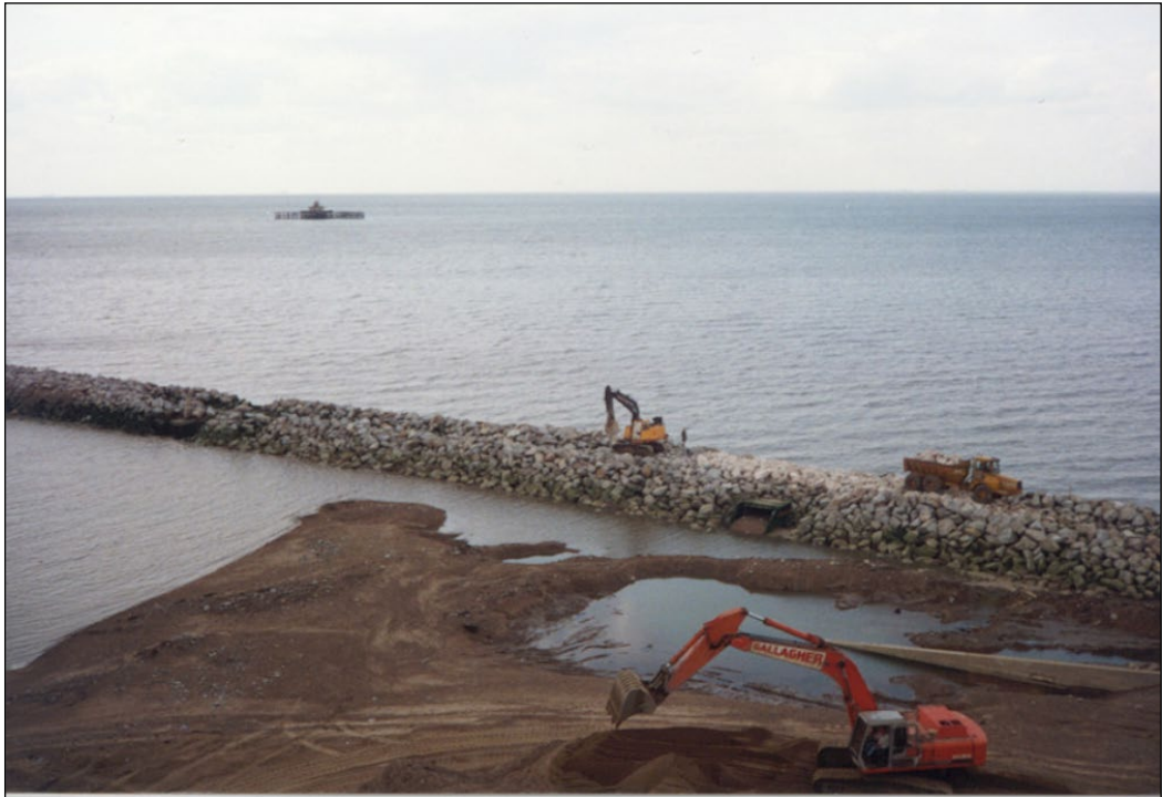
Figure 4.8 - Sea defences under construction at Herne Bay in 1990.
