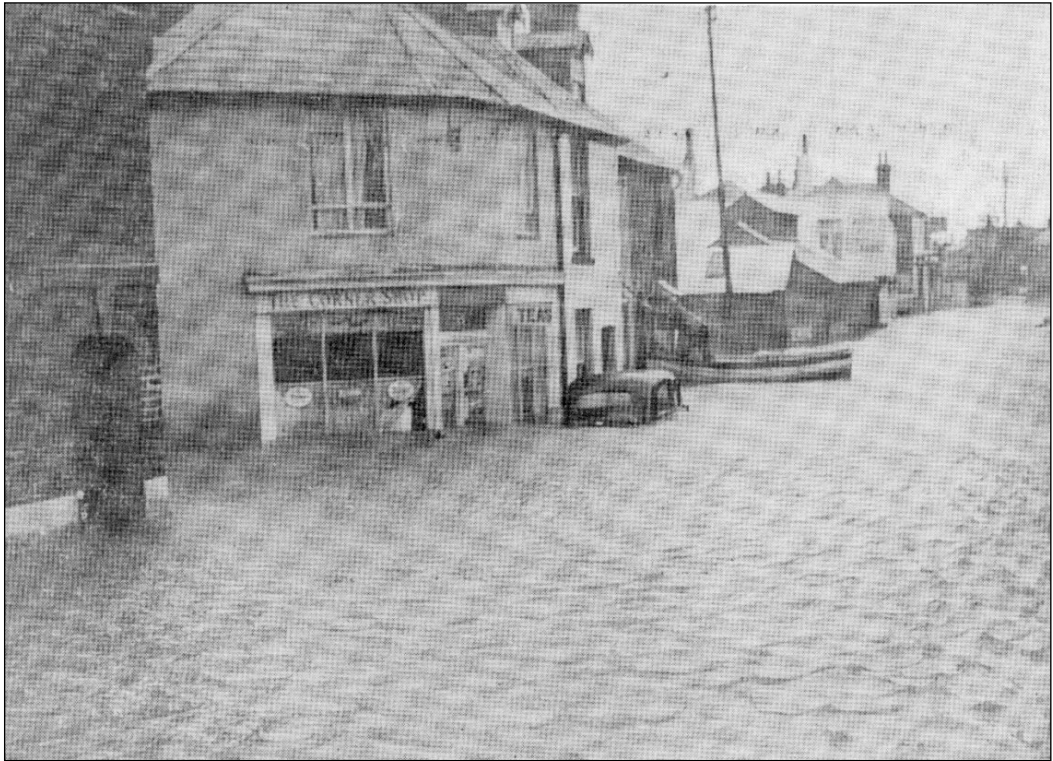
Figure 4.2 - Flooding at Whitstable, January 1953.
