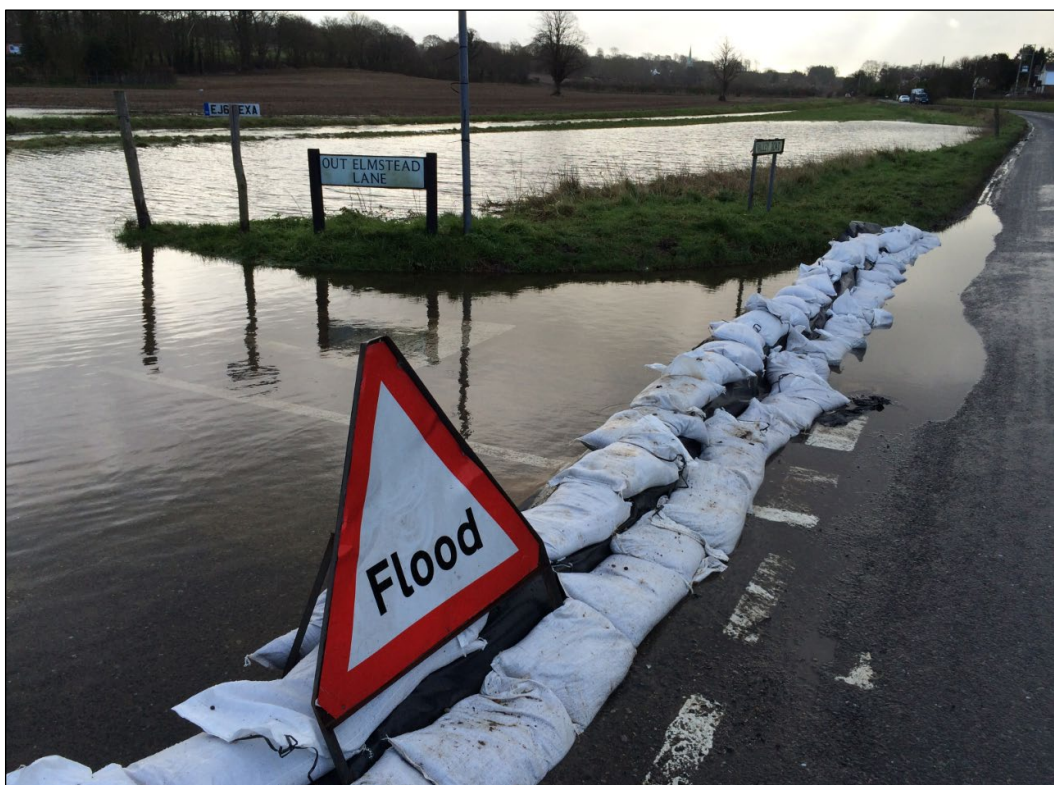
Figure 4.6 - Photograph of flooding at Out Elmstead Lane, Barham January 2014.
