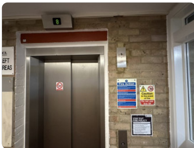
Fire Protection (Photo 17)
