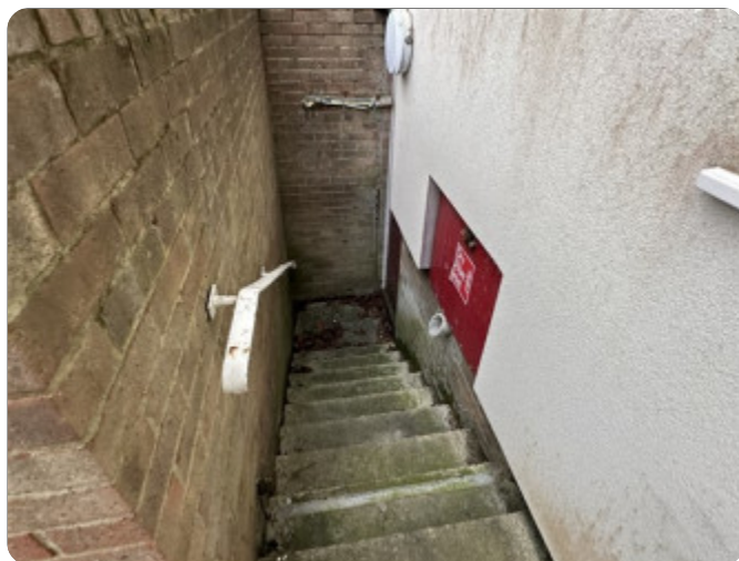
External Building Photo (Photo 6)
