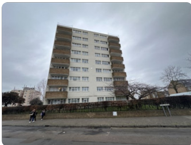
External Building Photo (Photo 1)
