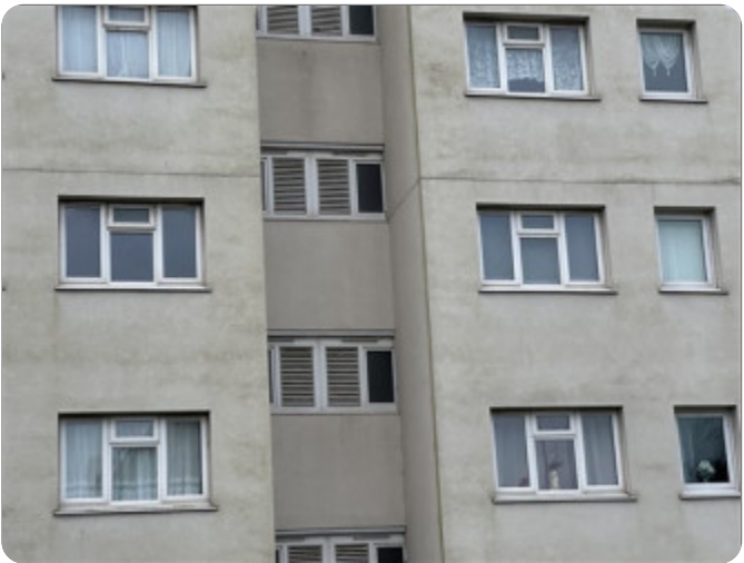
Fire Protection (Photo 9)
