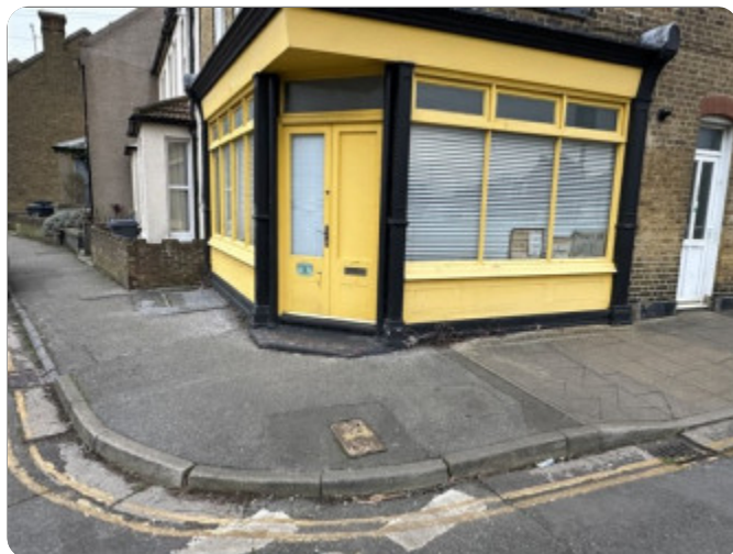
Fire Protection (Photo 3)
