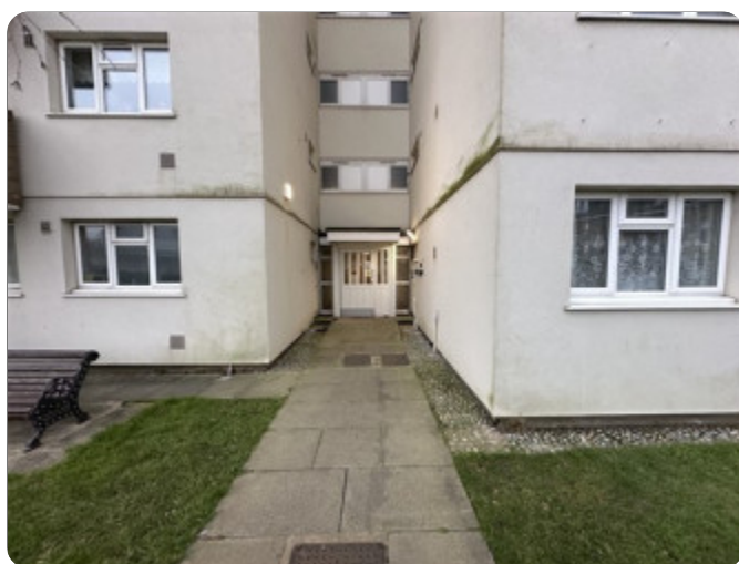
External Building Photo (Photo 3)
