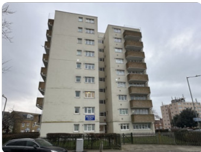
External Building Photo (Photo 2)
