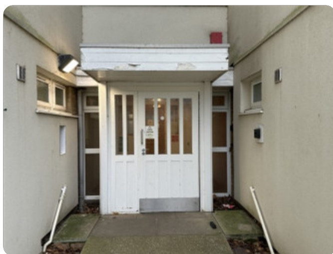
External Building Photo (Photo 4)
