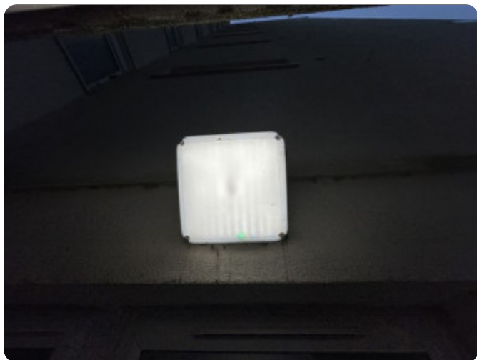
Fire Protection (Photo 2)
