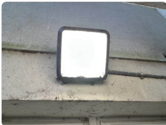
Fire Protection (Photo 7)
