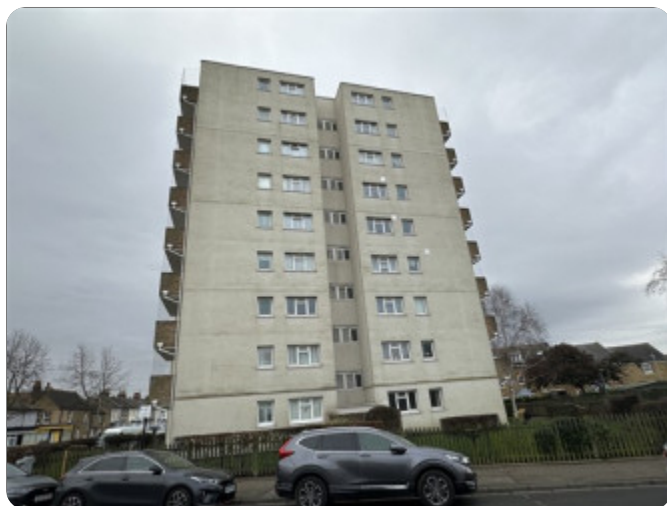
External Building Photo (Photo 5)
