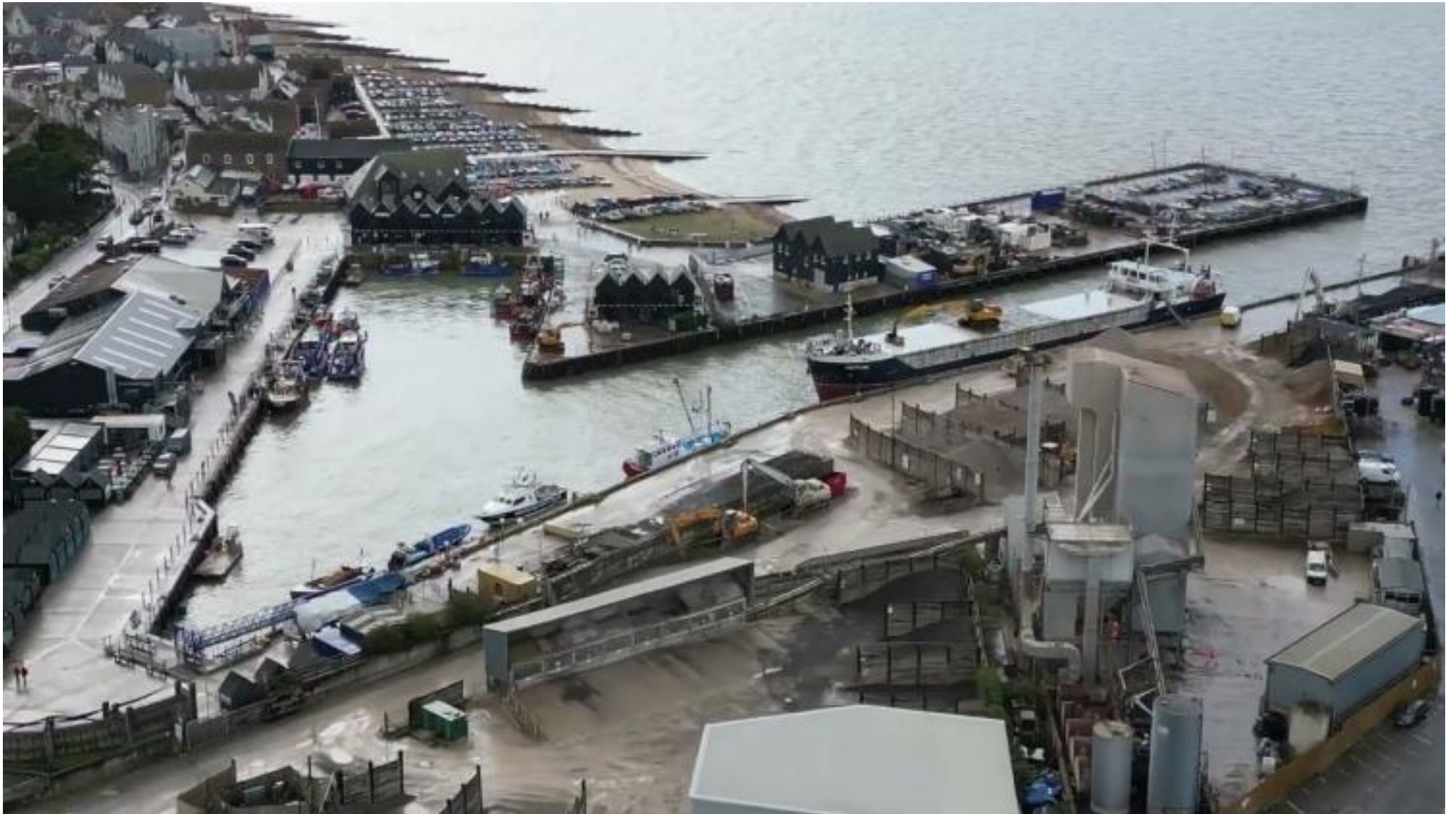
Aerial View of Whitstable Harbour Showing Ship Berthing Position
