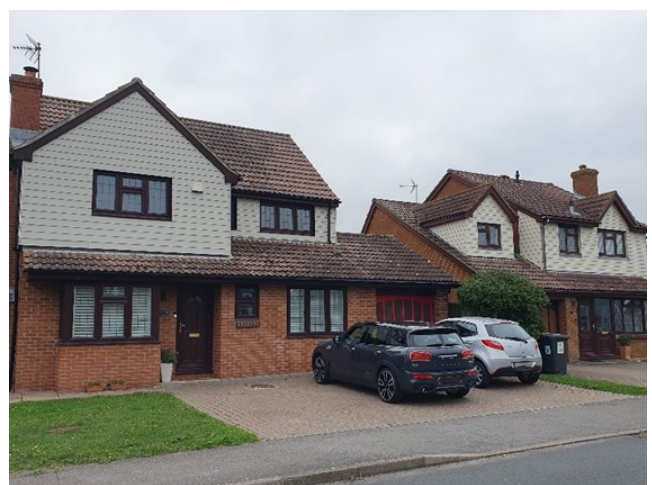
Figure 9 - Different styles in same estate reduces uniformity despite similar materials and colours. The varied roof lines help break the uniformity.
