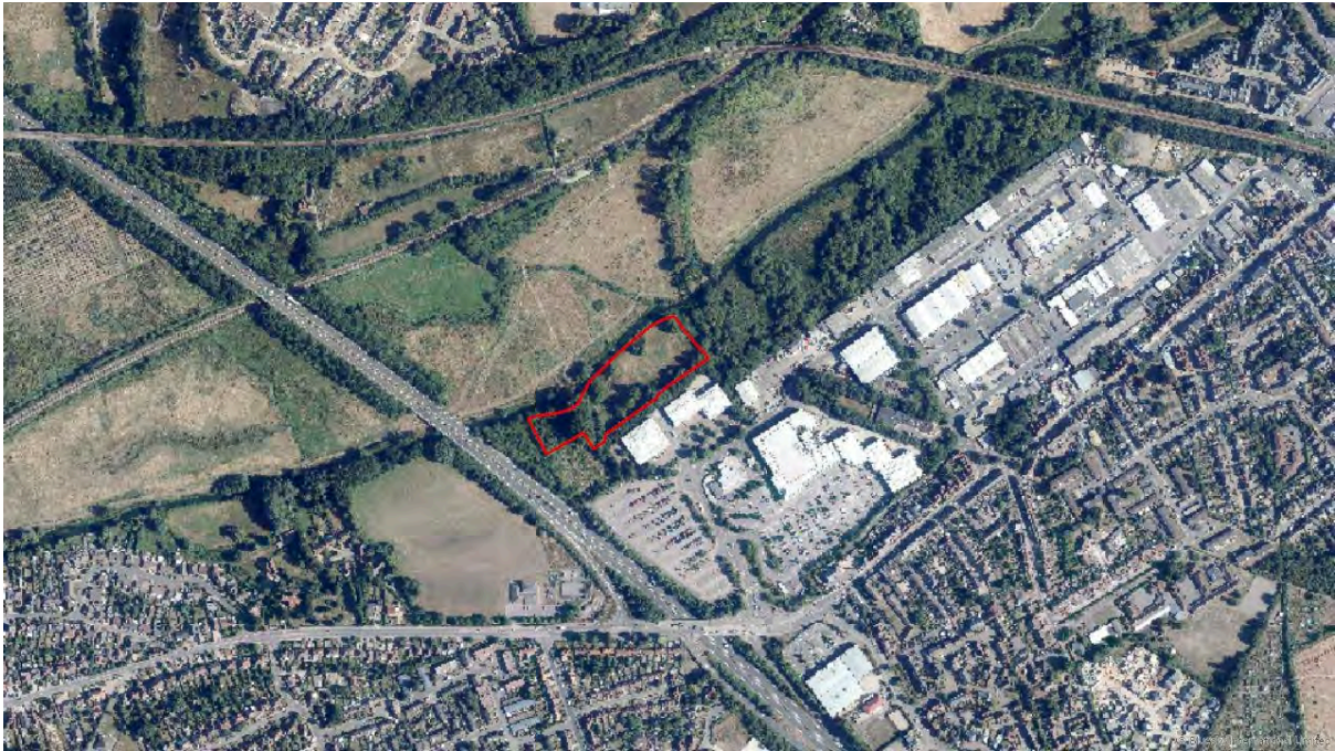
Figure D.1: Aerial photograph of Wincheap Meadow, Canterbury
