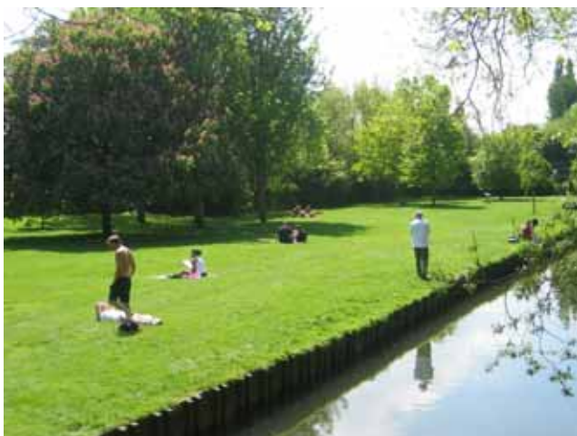
Before removal of vertical timber edge
