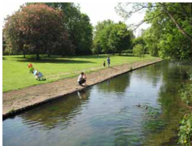
Timber edge removed and bank regraded
