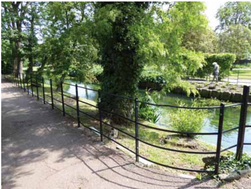
Typical paddock style railings used in parks and open spaces in the city
