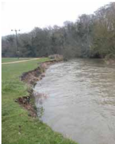
Natural erosion could, in time, interfere with Great Stour Way shared use path
